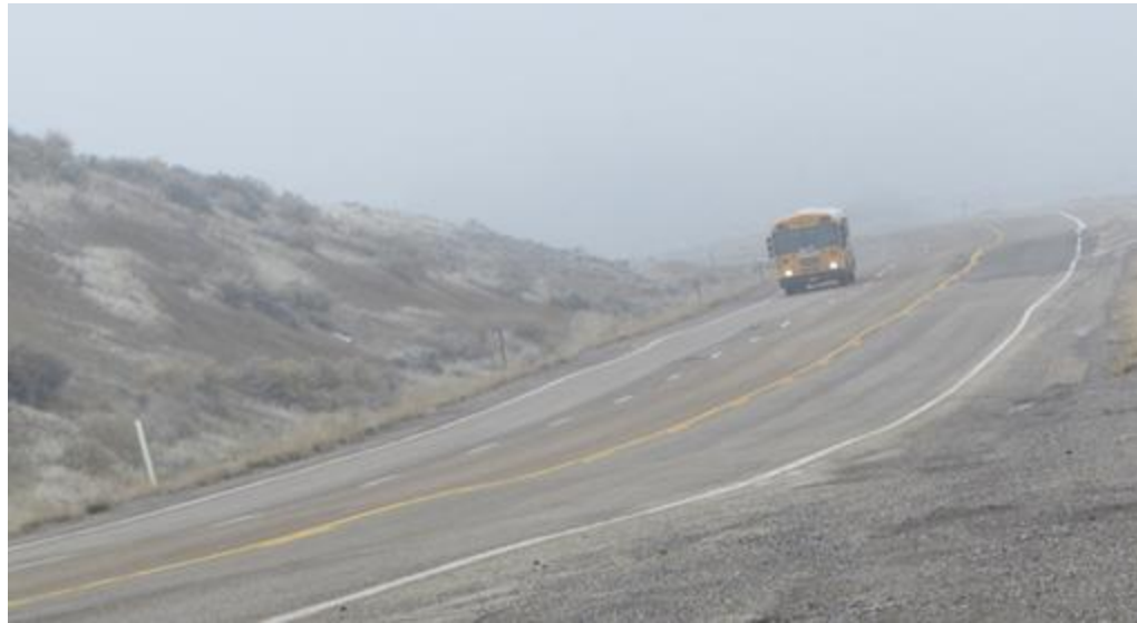
Figure 3.4 Problematic Sections of MP 16.3 to MP 18.0 (Picture Taken in May 2015)
